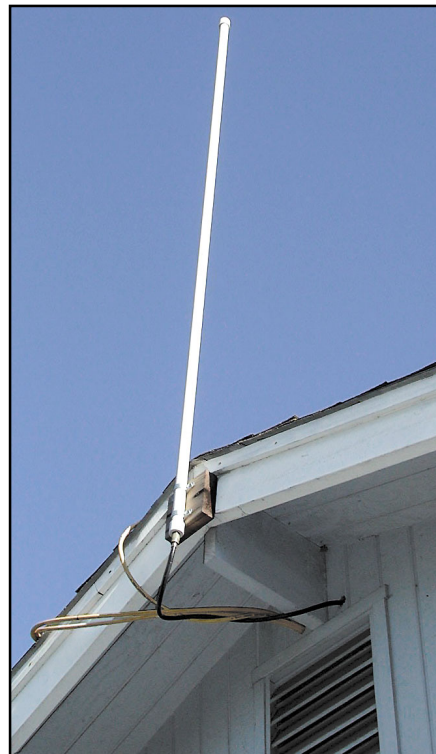
Figure 5—The completed antenna mounted to the roof.
