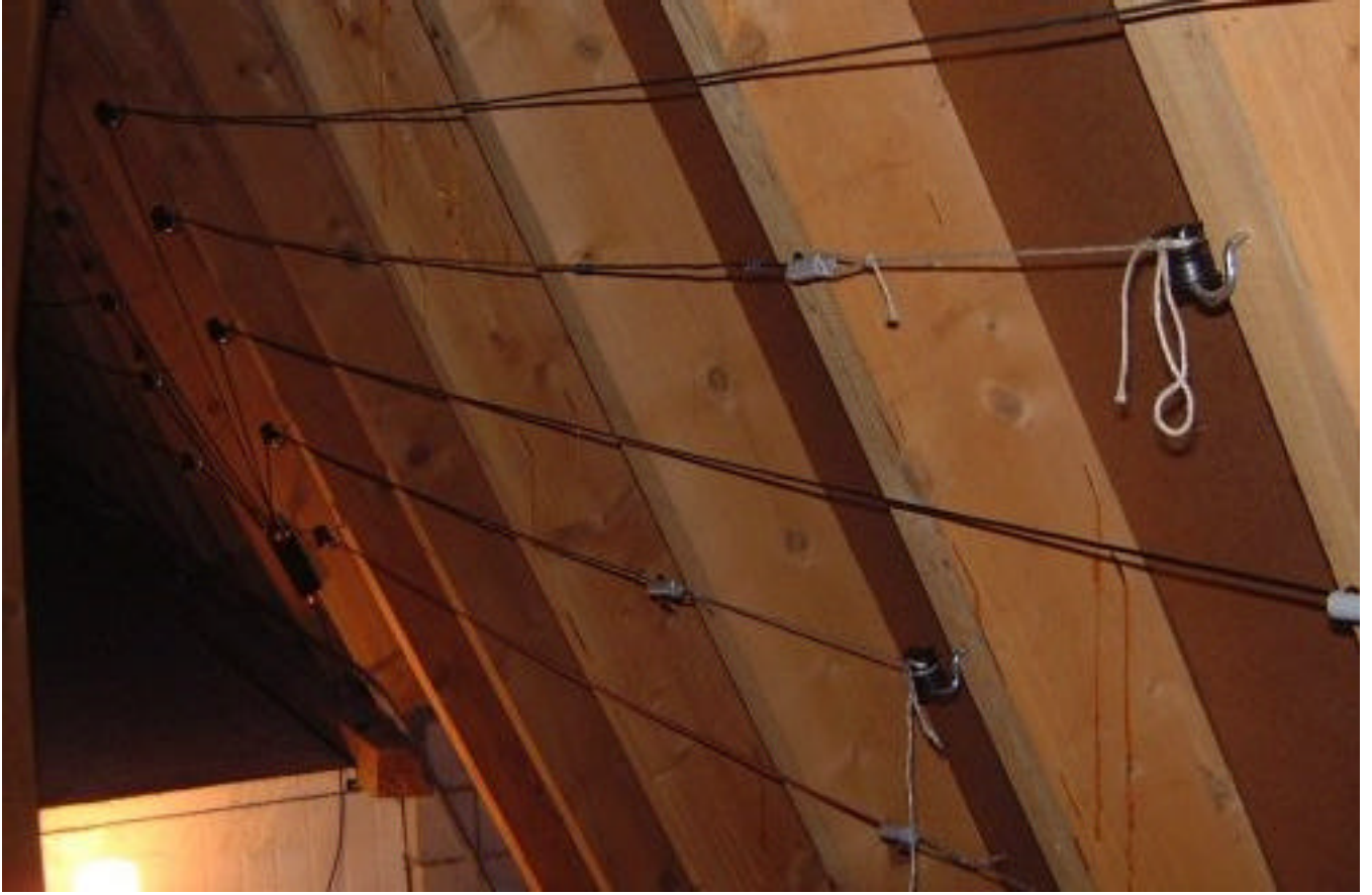
Antenna wires attached to roofspars Spacing between wires = 0.2m, spacing between roofspars = 0.6m
