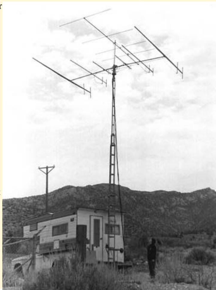
**Note:** All lengths are gross lengths. See text and photos for construction technique and recommended overlap at loop junctions. All loops are made of no. 18 AWG solid-covered copper bell wire. The Yagi-type directors are 1/16-in. brass brazing rod. See text for a discussion of director taper.
